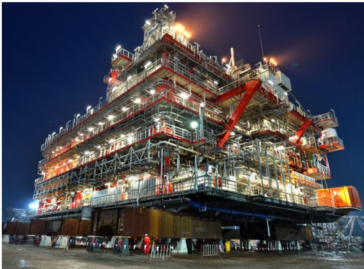
The topsides for the Gudrun project in the North Sea, a joint venture between Statoil and ENGIE (formerly GDF SUEZ). (Photo courtesy of Statoil / ENGIE.)
